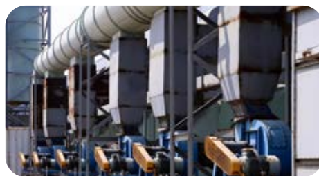
Dust bags Collection System and Integrated Waste Gas Treatment Device
